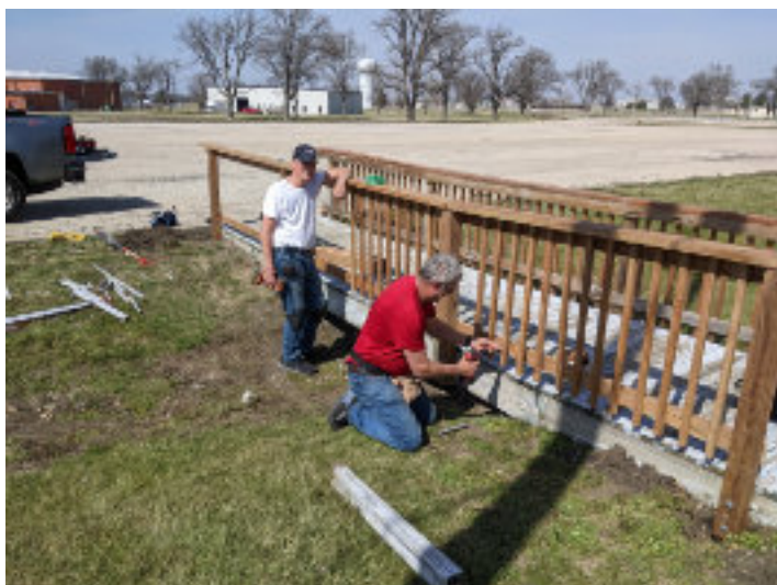
The Fix-It Friday team repairing the bridge (K. Drewelow photo)
